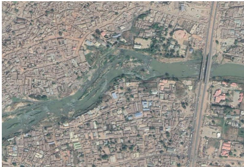
Plate 10: A typical Flood Prone Area in Gwagwalada
