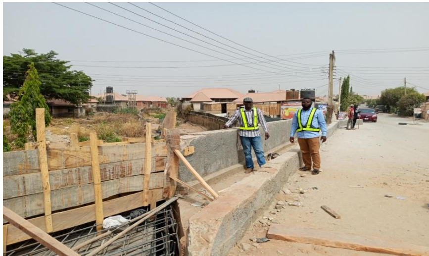
Plate 5: Trademore Bridge under re-construction caused by Flood
