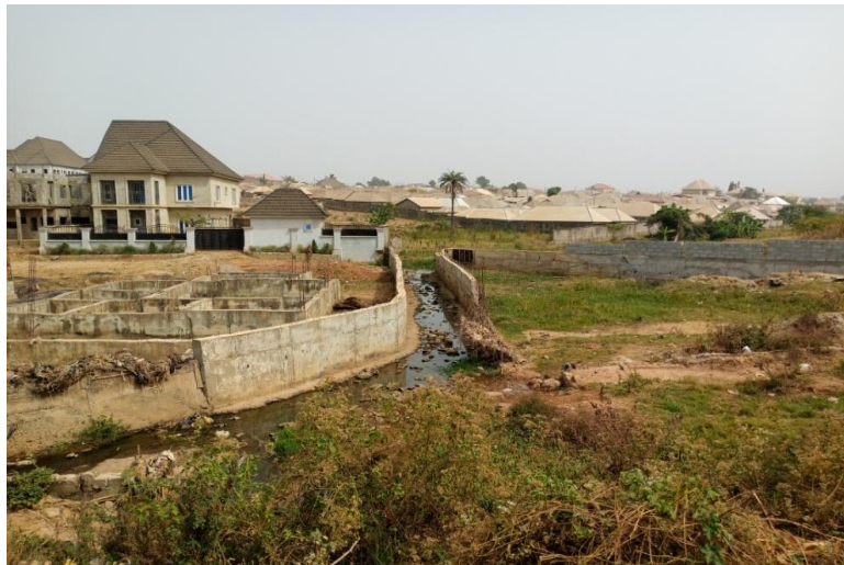
Plate 8: Buildings along the flood prone areas at Galadimawa
