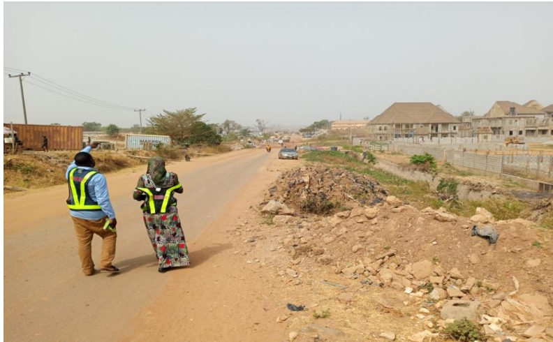
Plate 9: Part of Galadimawa with poor drainage system
