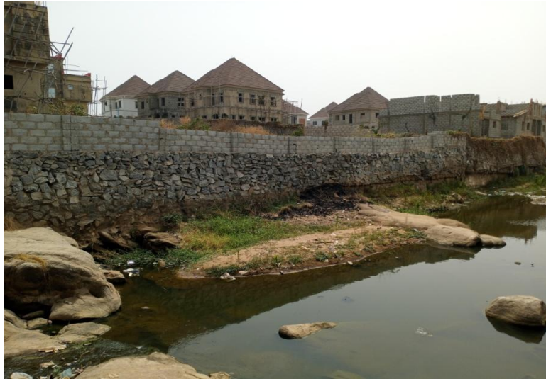
Plate 7: Flood Retention wall at Trademore Estate
