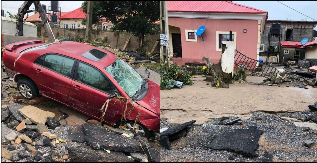
Plate 2: Effects of Flood on Road and Buildings
