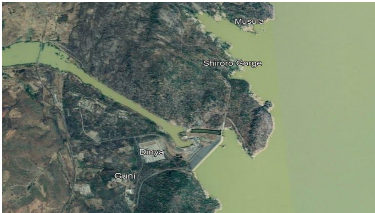
Figure 14: Detailed View Of Shiroro Dam
