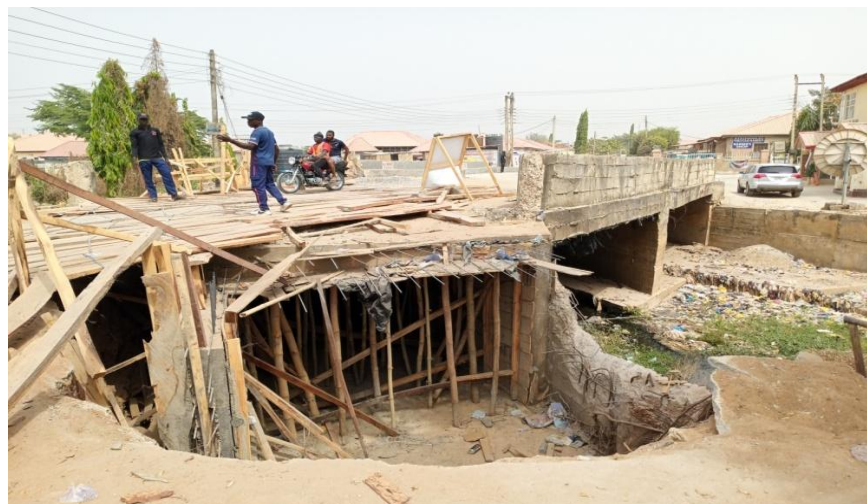
Plate 6: Trademore Bridge under re-construction caused by Flood
