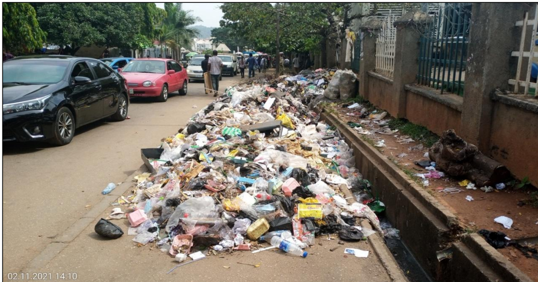
Plate 1: Drainage Blockage in Urban areas
