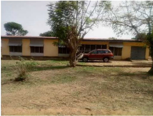
Plate 4: Case Study1 South Elevation Source: Fieldwork (2023)
