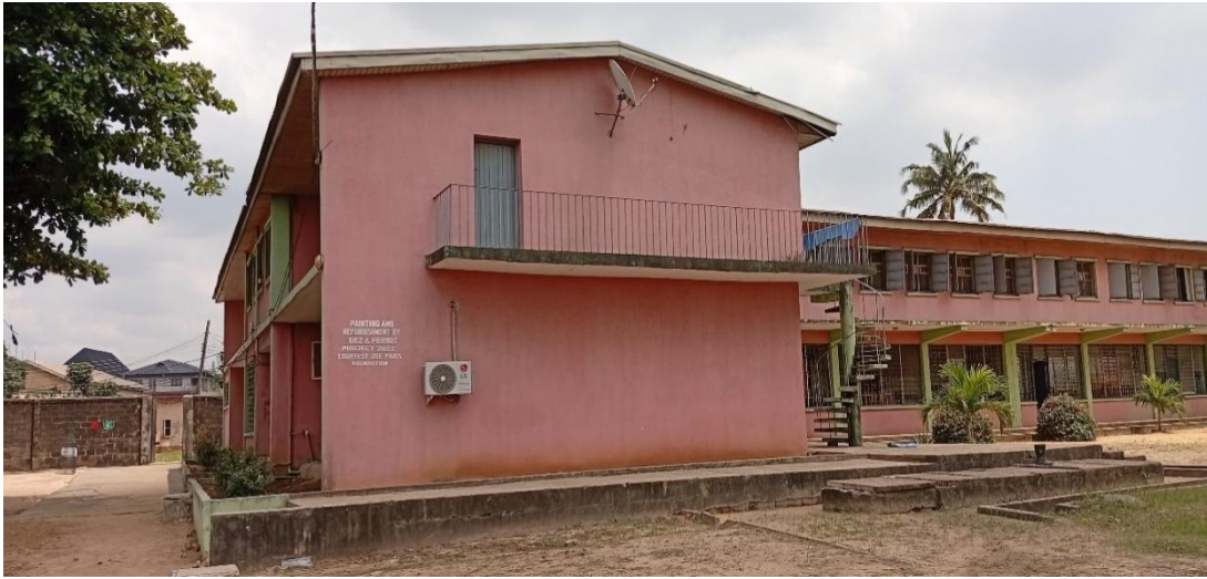
Plate 1: Oblique approach view into the facility compound Source: Fieldwork (2025)
