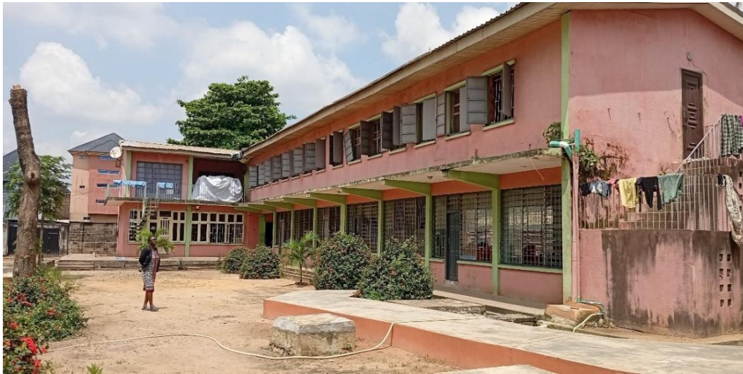
Plate 2: Right-hand view of the facility showing windows of dormitory on upper floor and workshops for vocational studies on the ground floor Source: Fieldwork (2025)
