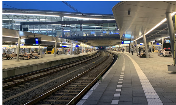
Figure 12: Showing Platform and Track Area
