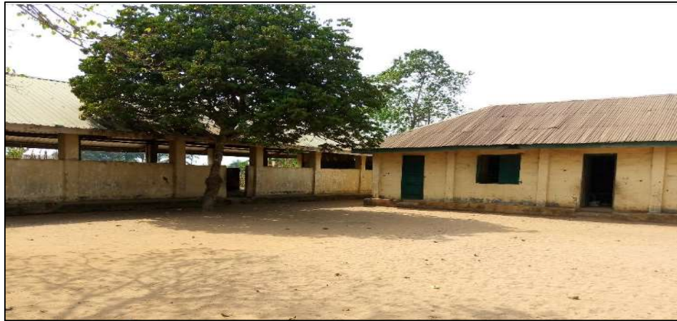
Figure 4: Sample school view showing 'dwarf wall' classroom (left side) and classroom with 'enclosed wall' classroom (right side) Source: Fieldwork, 2015
