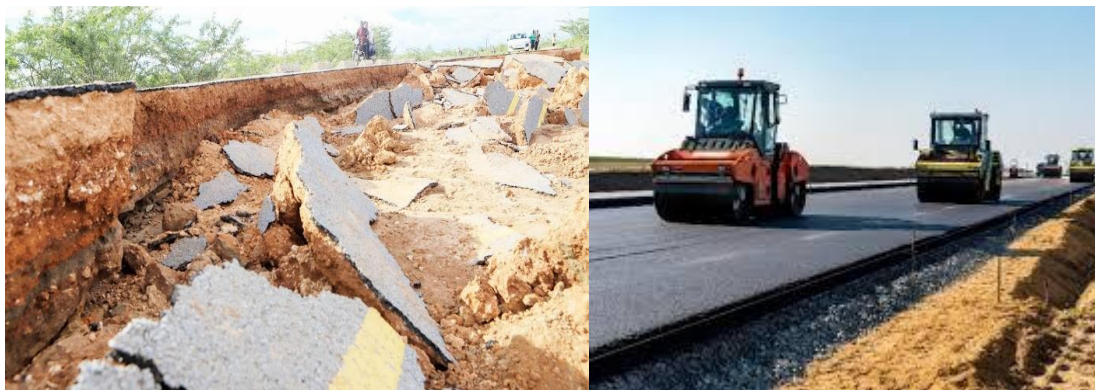
Plate 1: Dilapidated Road versus an ongoing road construction designed for resilience
