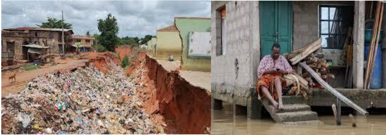
Plate 3: vulnerabilities arising from poor infrastructure
