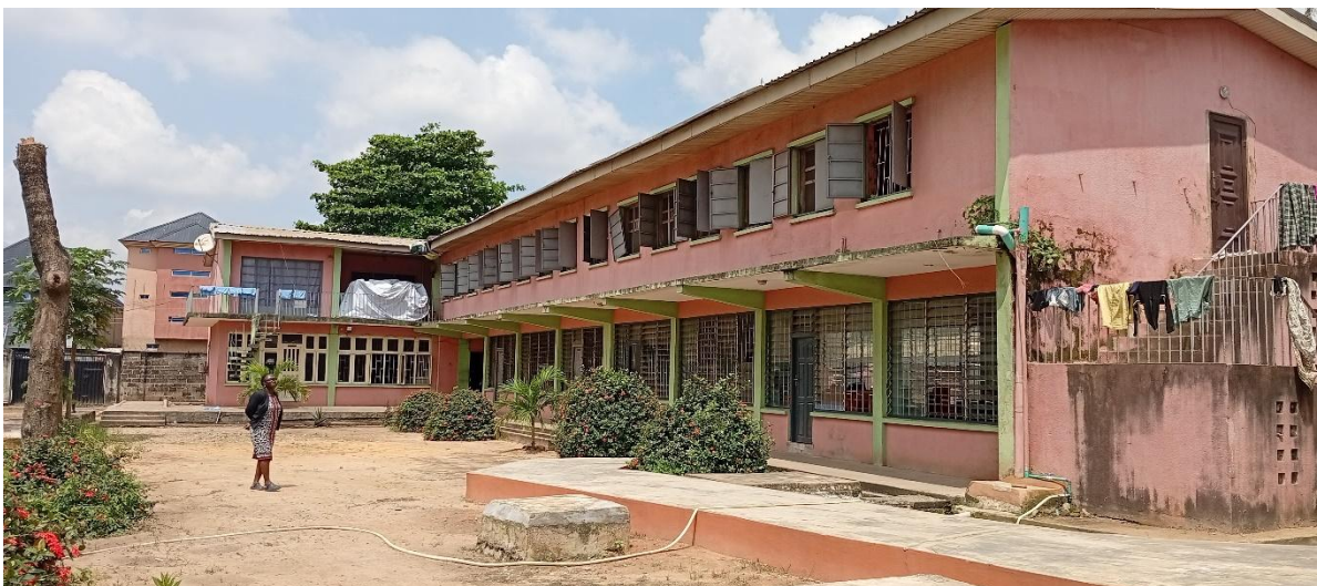
Plate 3: Right-hand view of the facility showing windows of dormitory on upper floor and workshops for vocational studies on ground floor
