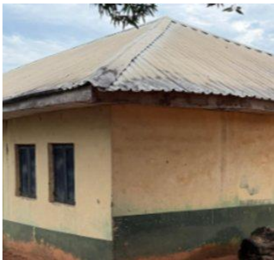
(a) SCB classroom — casement window system
