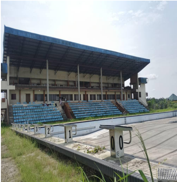
Plate 1: Outdoor seating area facing the swimming pool
