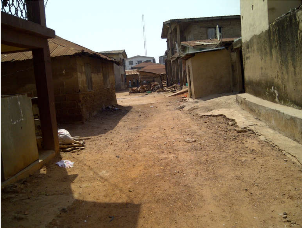
Figure 4: Typical family house built with laterite and zinc roofing sheet
