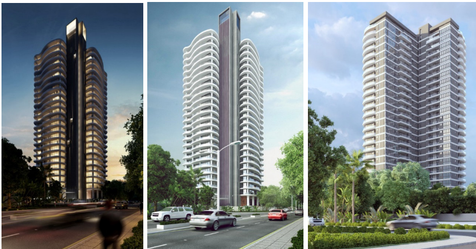
Figure 8: The Tower at #4 Bourdillon Drive – Ikoyi, Lagos
