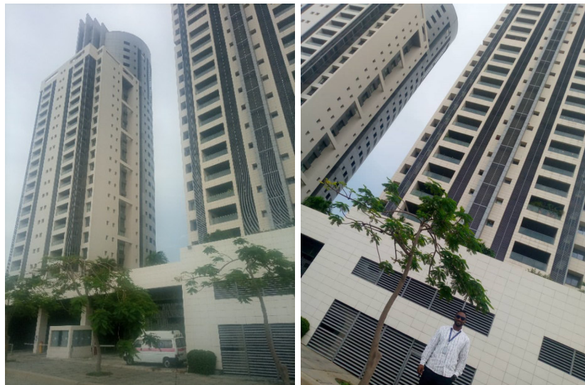
Figure 4: Champagne Pearl (Right) and Black Pearl (left) Towers, Victoria Island, Lagos
